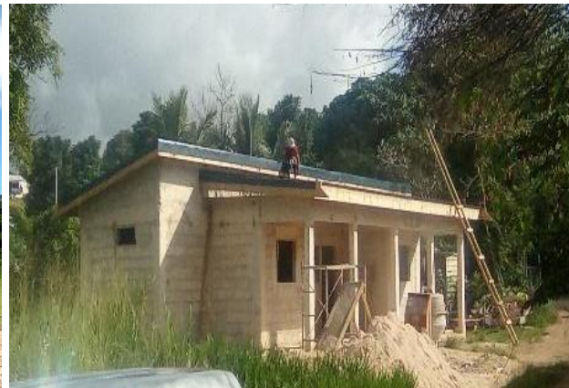
Sanma DoWR Laboratory Building in Progress
