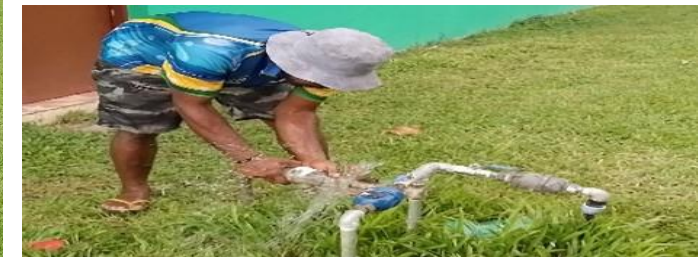
Replacing Damaged / Faulty Metres
