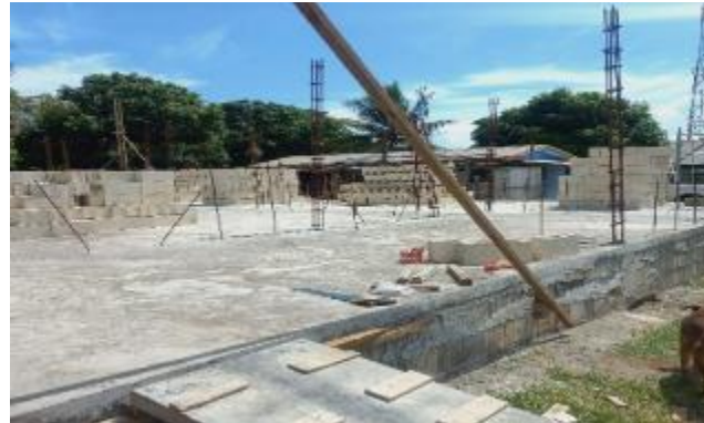
Penama / Saratama DoWR New Office Building in progress
