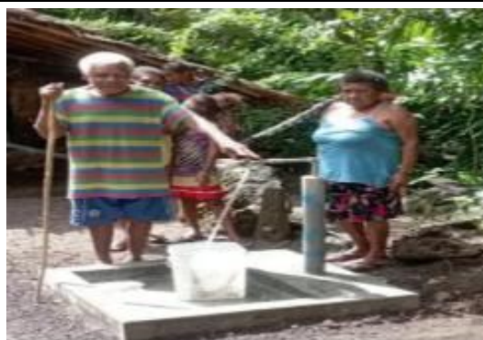
Mota Water System Complete
