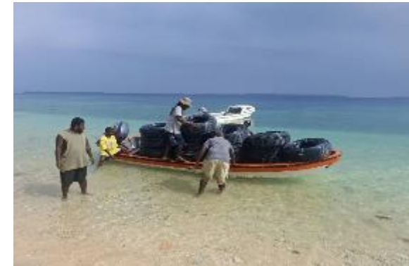
Drilling team completing new bores by shipping Pipes to Tutuba
