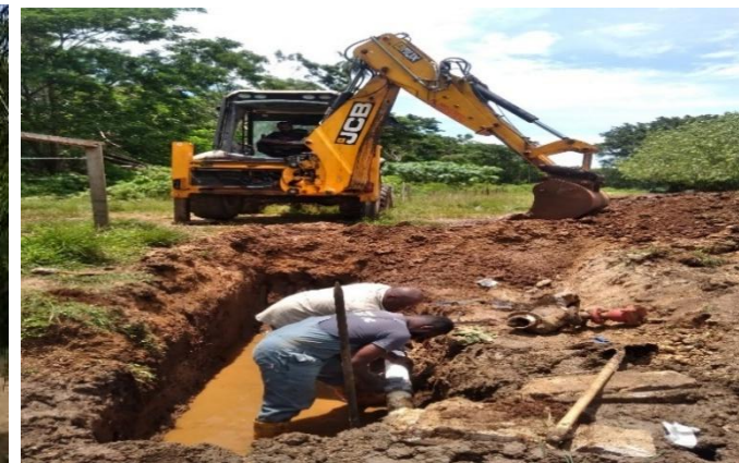
Repaired main pipe 100mm ground PVC to showground
