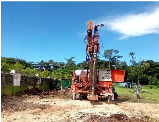
DoWR Drilling Team in Progress
