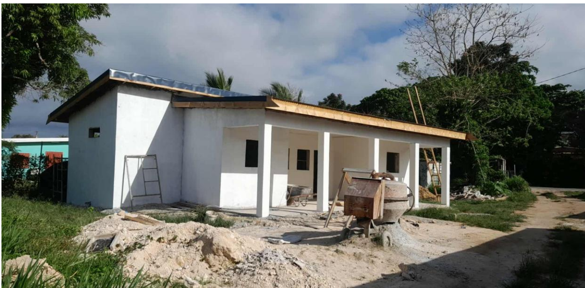
DoWR Sanma Laboratory Building Construction in progress
