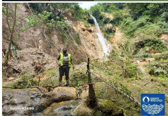
Evaluation of the Mele Source Damage Following the Earthquake
